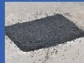
Temporary Asphalt Repair
