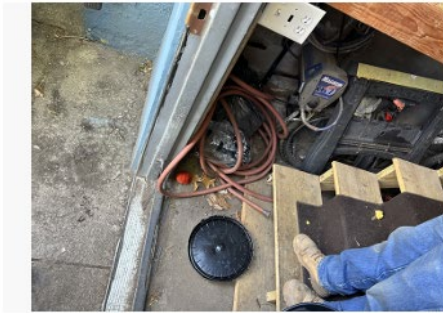
D52A70F9-22BC-491C-9A41-AC1DDCEB73EC-10899-000004AAADE09035.jpeg - SI_12_Interior - Preconstruction
