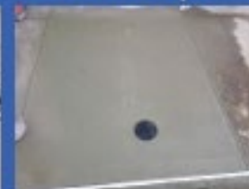
Permanent Sidewalk Repair
