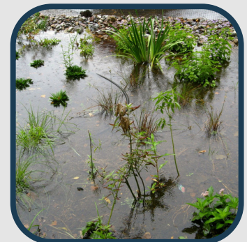
Stormwater enters the Berkeley Hts garden at the top.
