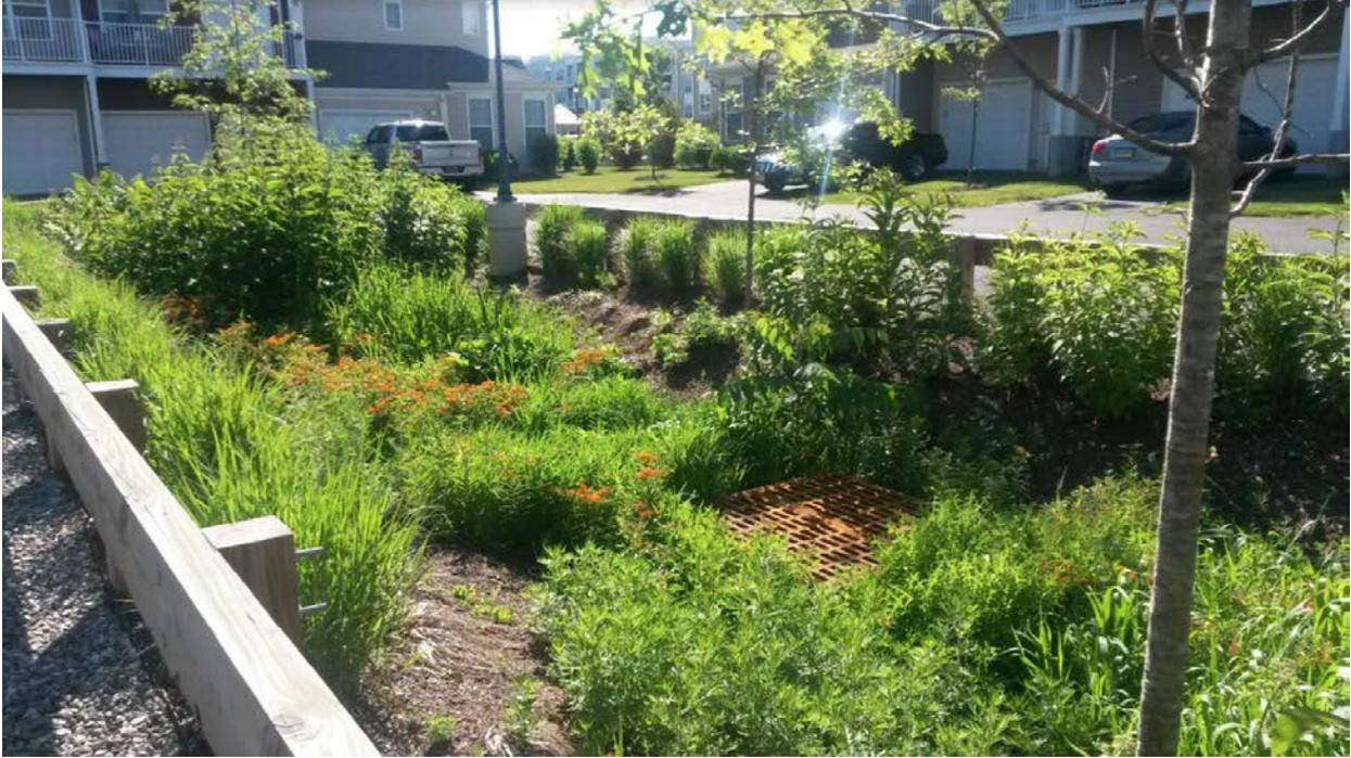
*Stormwater utilities support the development of green infrastructure to manage stormwater, like this bioretention system in Somerset, NJ. Source: Maser Consulting, 2020.*
