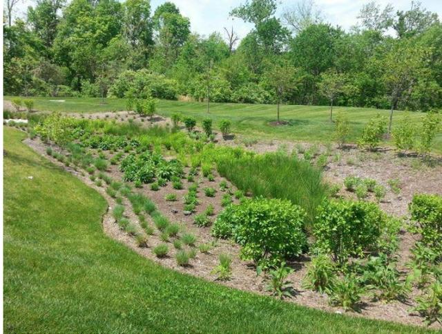
*This new bioretention basin will help manage stormwater on-site. The development of stormwater utilities can help encourage this and other green infrastructure practices. Source: Bluegrass Landscape and Maintenance, 2018.*
