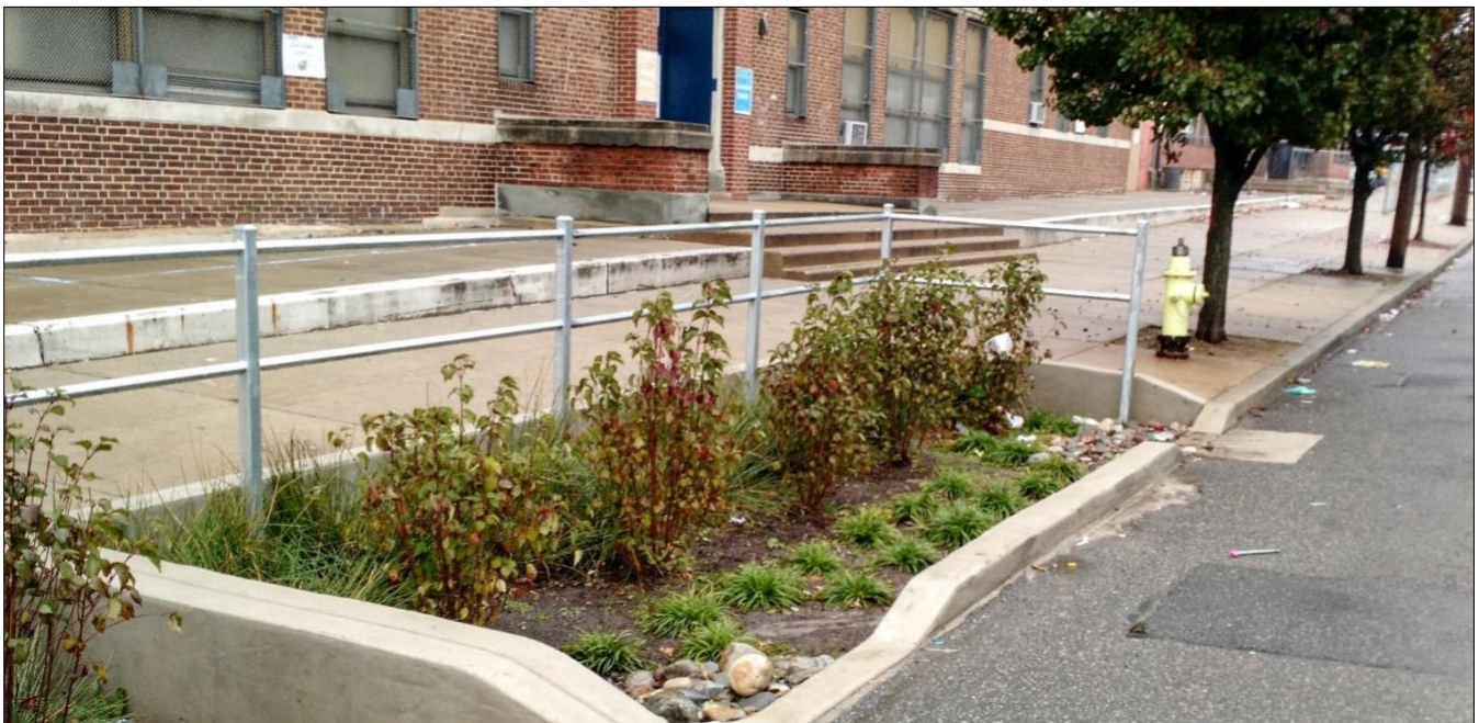
Figure 2. Bonsall School stormwater planters in Camden, NJ. Credit: Camden County Municipal Utilities Authority
