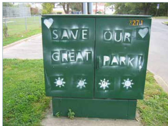
This decorated utility box in Von Neida Park shows neighbors’ awareness of the need to create a healthy park.
